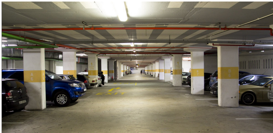
Figure 5.1: Representative picture of an indoor parking facility showcasing alphanumeric markings on pillars, serving as parking spot identifiers.
