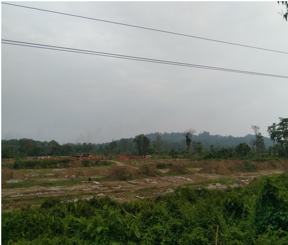
Brickkiln site near Ongsa Village, Kharsang, run by a non-local contractor
