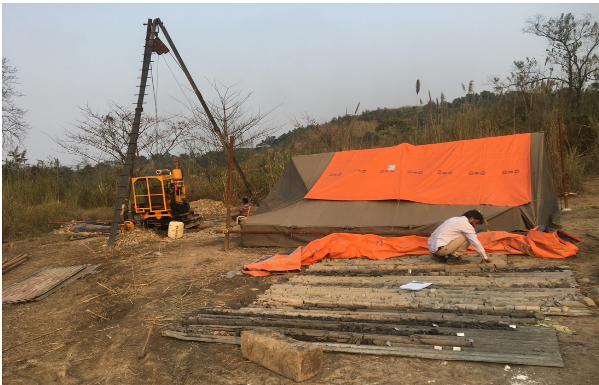
Coal survey site near Longsi village
