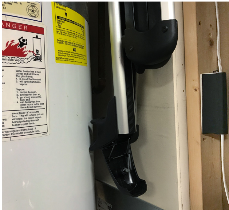
Figure 5-10: A possible implementation of a temperature monitor deployed on a stud (location E)
